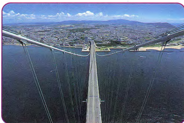
Japan's Akashi-Kaikyo Bridge is the longest suspension bridge in the world.
