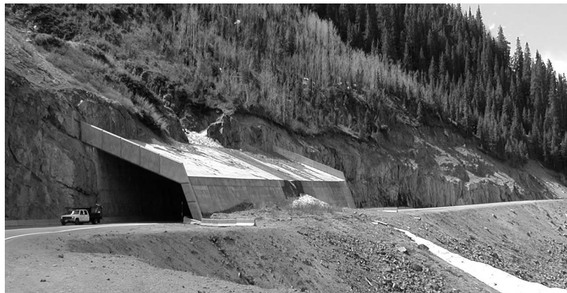
Figure 9-8 This snow shed in the Rocky Mountains protects the road and people who travel on it from avalanches and landslides.
