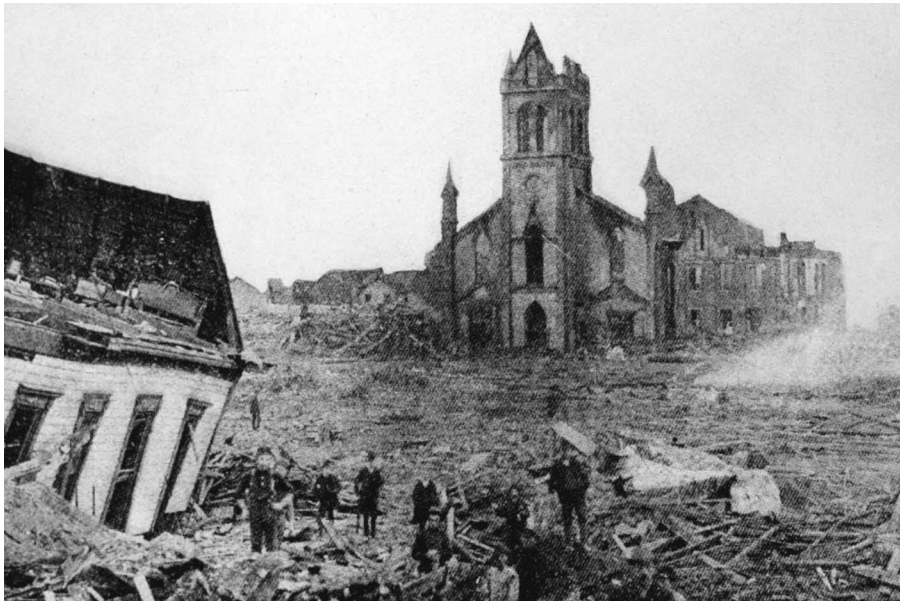
Figure 23-1 Damage caused by the 1900 Galveston Hurricane.
