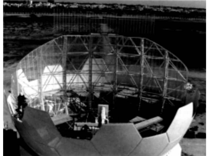
Figure R11 ASR-23SS radar antenna (Raytheon Company photo).
