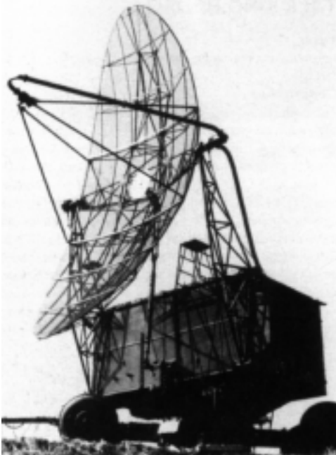
Figure R30 A Russian S-band nodding height-finder radar (from Jane's, 1995, p. 49).
